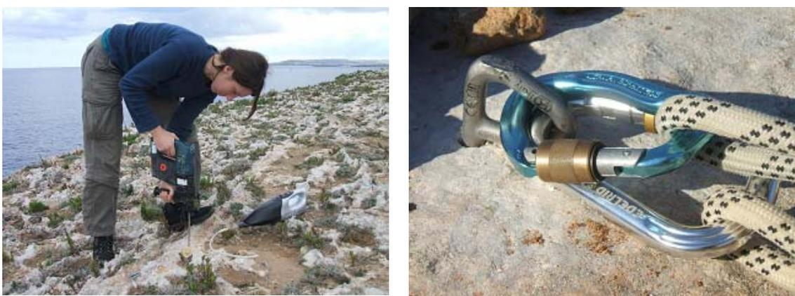
**Figure 2: Fixing the climbing bolts.** Holes were drilled into the rock with an HSS drill, using a small vacuum cleaner to extract dust from the holes. The glue was left to set for 24 hours before use.
